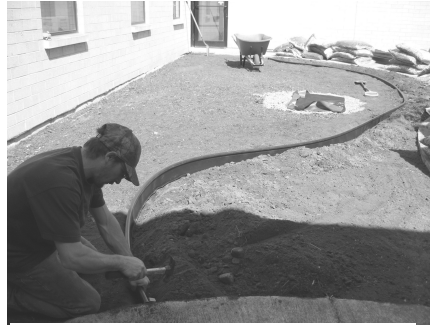
Doug Rehwinkel lays path edging.
